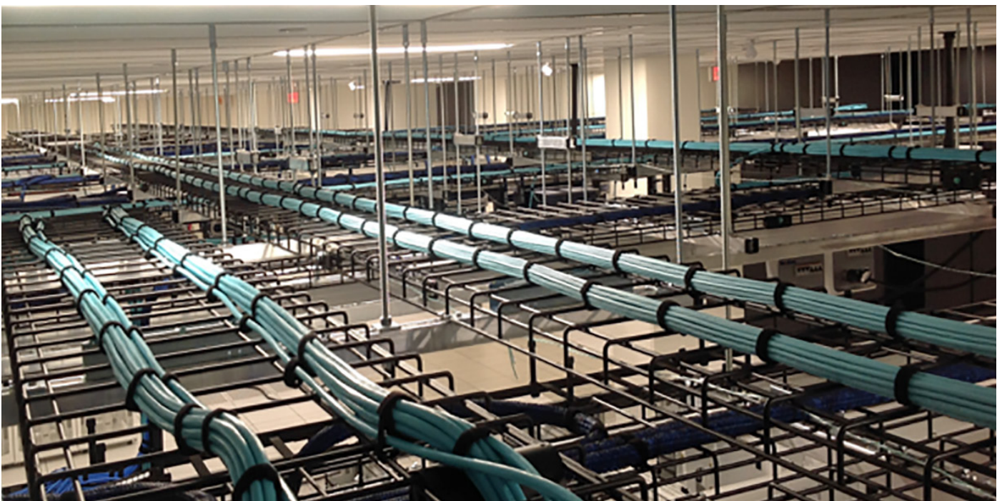
FIGURE 10: Take note of the clean, professional cable dressing that is consistent throughout the POD.
